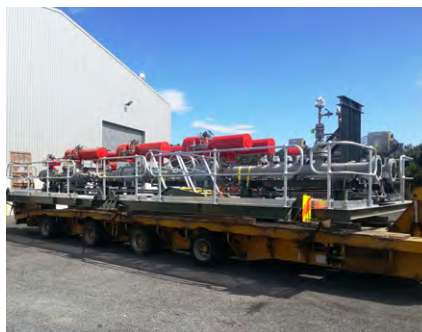
48 tonne Valve Module being lifted onto its piles. Left: The Valve Module leaving the EWL workshop. Below: The OPP Module leaving the EWL workshop.
